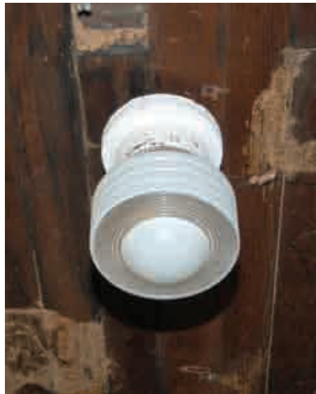
New lighting fixtures are a must in Busk’s renovated homes, as most have electrical systems that are worn out and substandard.
