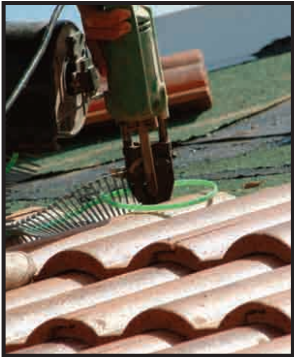
The rebuilt home featured storm-proof additions such as roof tiles attached with two stainless steel screws (left), enhanced metal roof connectors (top right), and solid wood blocking behind the soffits, shown prior to finishing (bottom center), and in finished form (far right).
